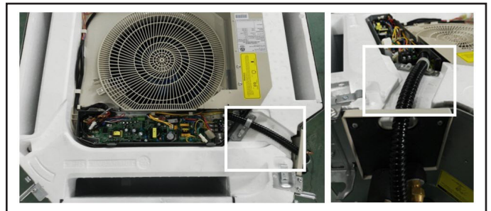
Figure 9. Field-Supplied Electrical Conduit Example
